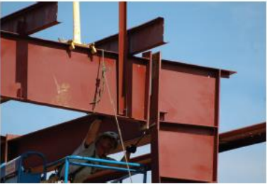
(b) Metal building (photo courtesy of MBMA)
