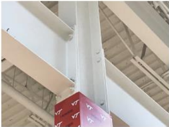
(a) Conventional steel building (photo from Matt Eatherton collection)
