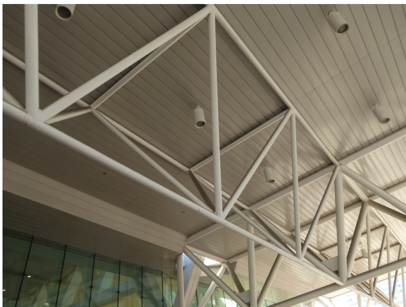
(b) Triangular truss with KK-connections
