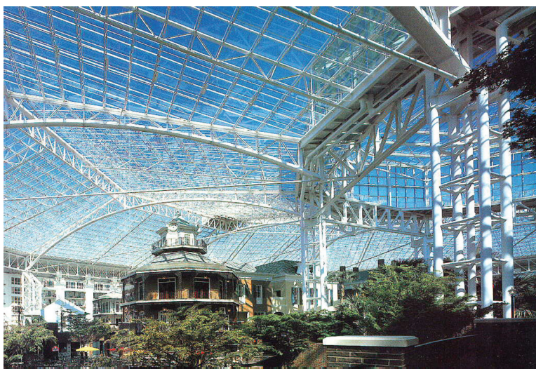
Fig. 1-5. Opryland Hotel, Nashville, Tennessee.
