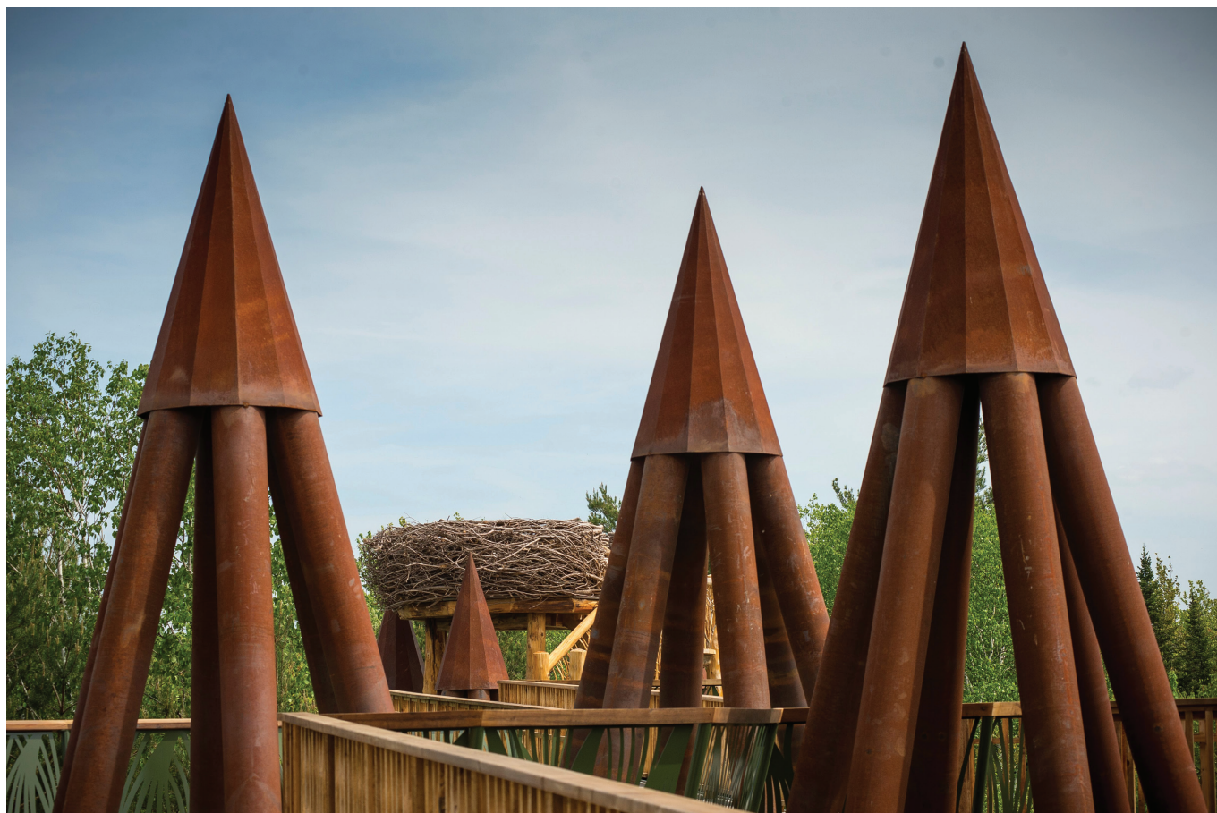
Fig. 1-13. ASTM A847/A847M weathering steel HSS (photo courtesy of The Wild Center, New York).
