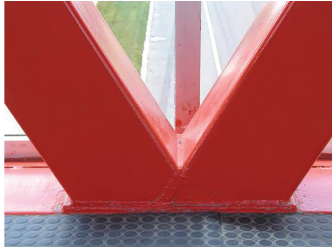
(b) Smooth surface finish with cold-formed HSS
