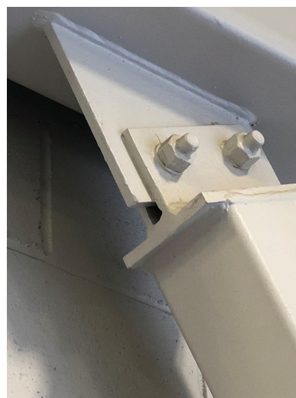
(b) Installed forked tee end connection
