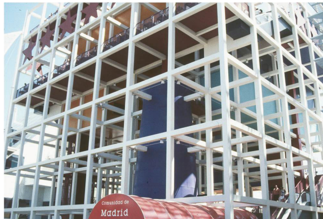
Fig. 3-10. 3D moment-resisting frame using equal-width HSS members.
