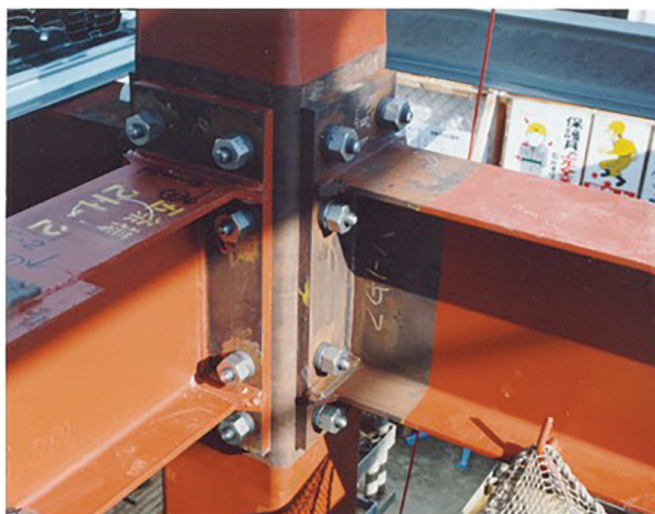
Fig. 4-8. Beam-to-column end-plate connection using blind bolts.
