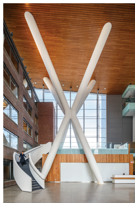
Fig. 1-10. Examples of large-size tubular columns to API specification (photos courtesy of Interior Images and Cast Connex Corporation).
