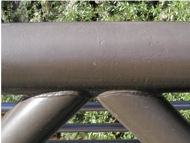
(a) Rough surface finish with hot-formed HSS
