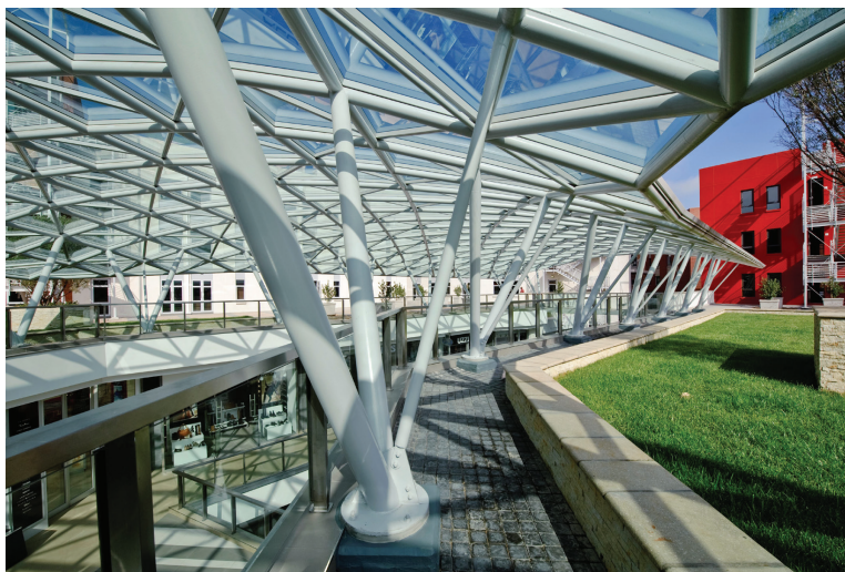
Fig. 1-6. Melrose Arch Galleria, Johannesburg, South Africa.
