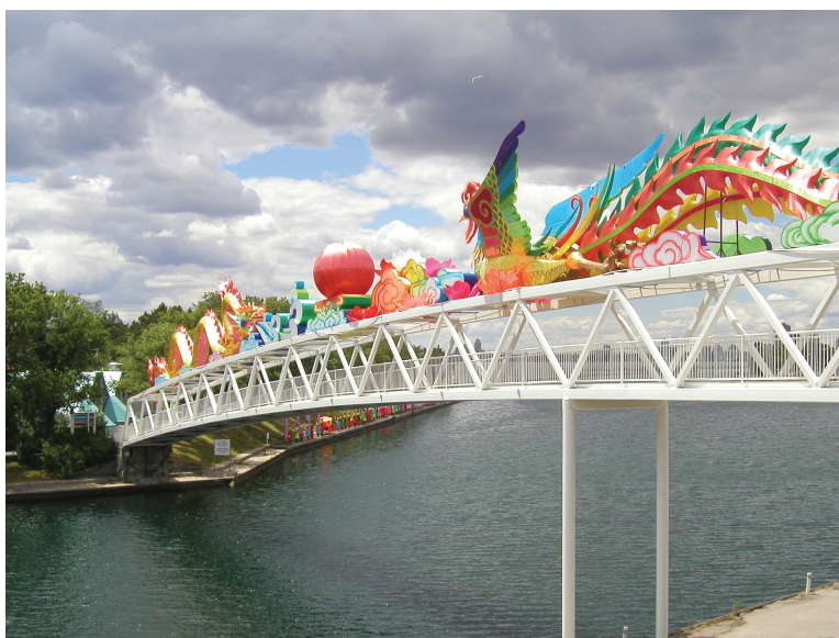
Fig. 1-4. Warren truss pedestrian bridge, Ontario Place, Toronto, Canada.
