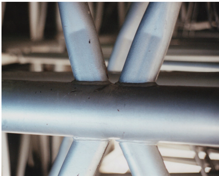
Fig. 3-15. Round-to-round HSS connection with end-flattened branches.
