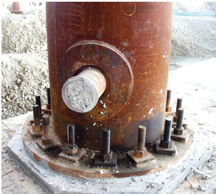
Fig. 1-14. Filling a round HSS by pumping concrete from the bottom of the column.
