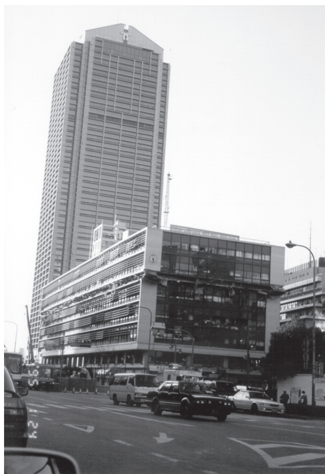
Fig. 1-7. Kobe City Hall (photo by M. Bruneau).
