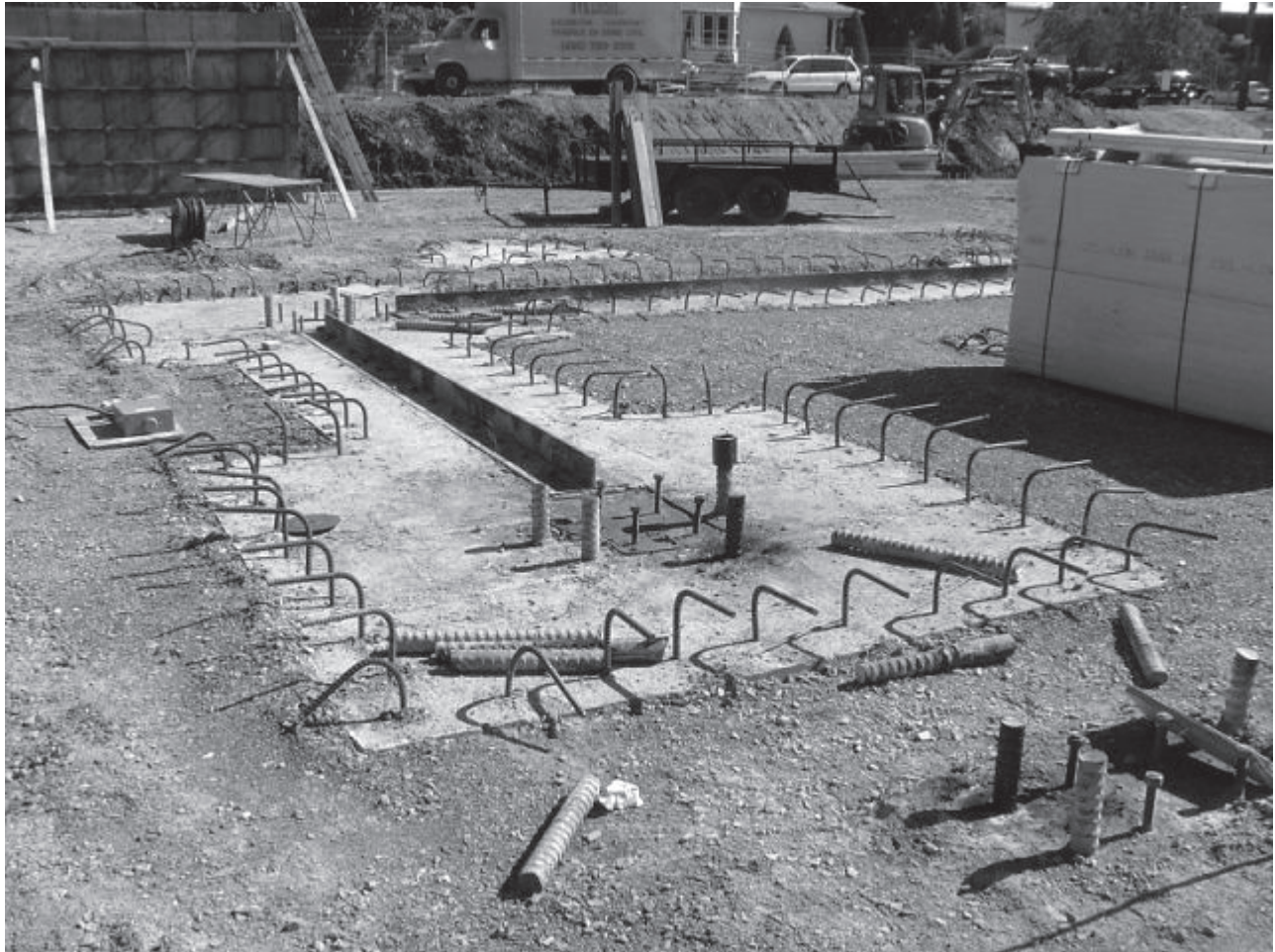
Fig. 1-33. SPW and details at base of SPW, ING building (courtesy of Louis Crepeau and Jean-Benoit Ducharme, Groupe Teknika, Montreal, Canada).
