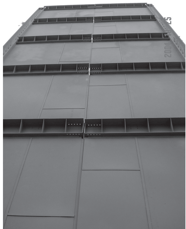
Fig. 1–32. Close-up view of wall at mid-span splice location, ING building (courtesy of Louis Crepeau and Jean-Benoit Ducharme, Groupe Teknika, Montreal, Canada).
