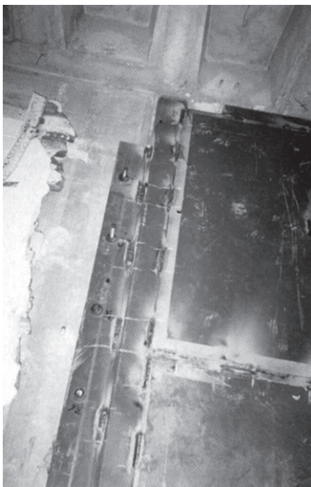
Fig. 1-18. New steel plate shear walls (courtesy of KPFF Consulting Engineers, Portland, OR).
