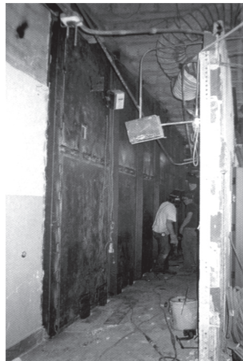
Fig. 1-17. Installation of new steel plate shear walls (courtesy of KPFF Consulting Engineers, Portland, OR).
