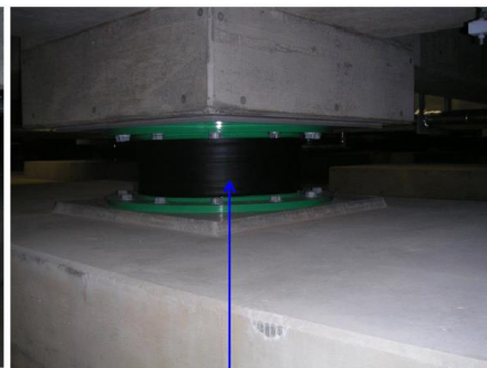
Natural rubber-laminated isolator (NRB)
